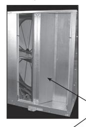
This panel must be removed before the energy wheel can slide out. (ERV-522 only)
